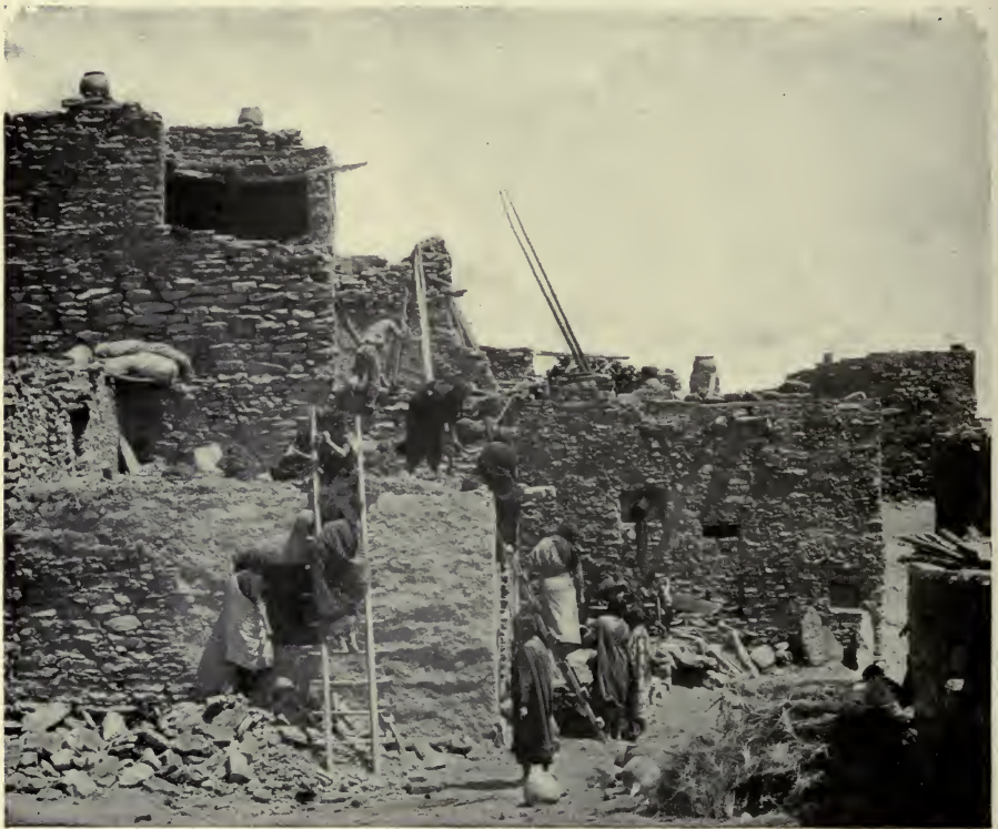
HOPÍ WOMEN BUILDING A HOUSE AT ORAIBI, ARIZONA.
